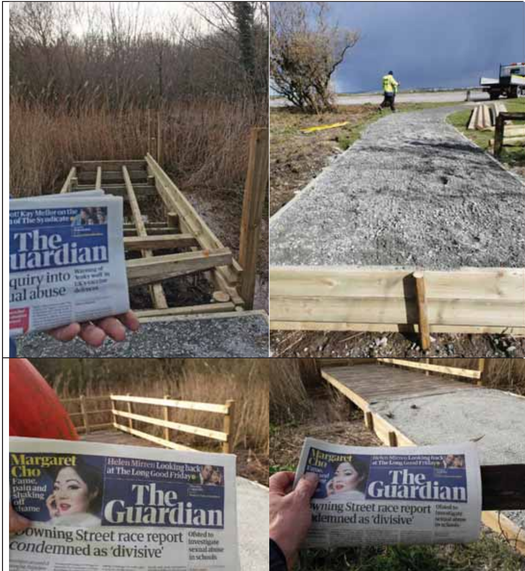
The above photographs confirm progress of work prior to 19 th April 2021
